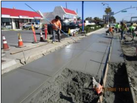
Finishing driveway north side of Carson.
