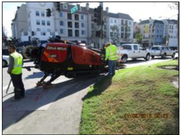
Directional boring for traffic signal conduit.
