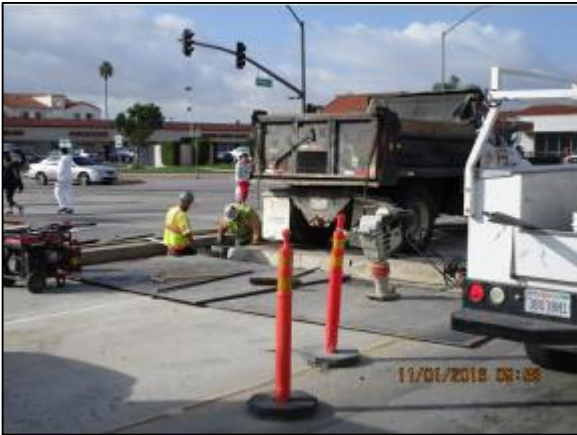
Excavating to locate water line.
