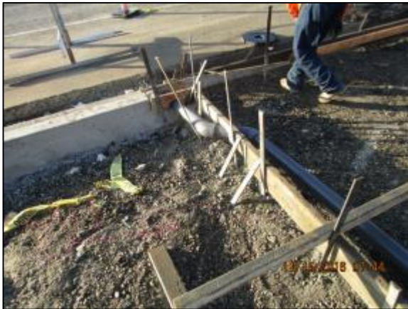
Installing drain under driveway.
