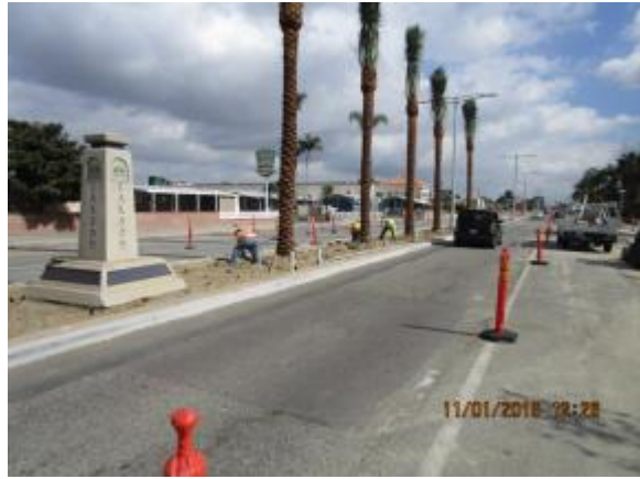
Forming curb and gutter.
