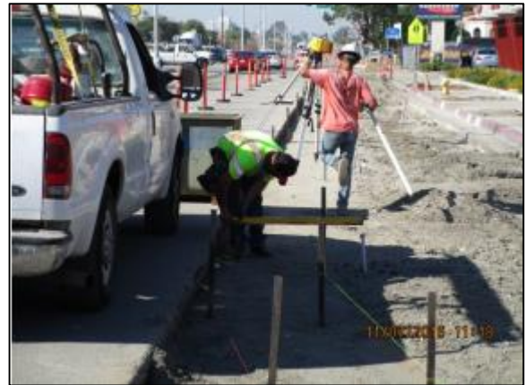
Forming curb and gutter on north side of Carson.
