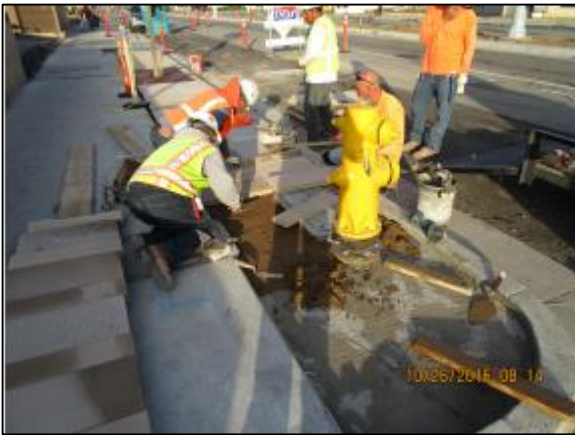
Placing Architectural Pavers
