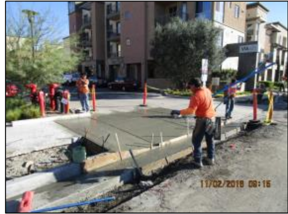
Placing driveway on north side of Carson east of Dolores.
