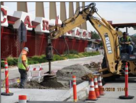
Auguring holes for F1 poles on north side of Carson.
