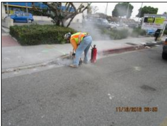
Saw cutting curb and gutter for driveway replacement.
