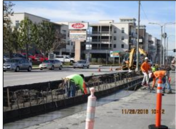
Placing curb and gutter on median island west of Avalon.
