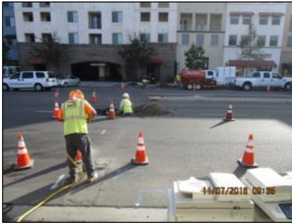
Potholing on Avalon for directional boring.
