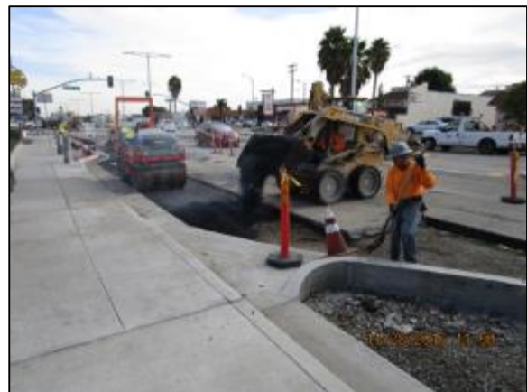
Paving slots on north side of Carson.
