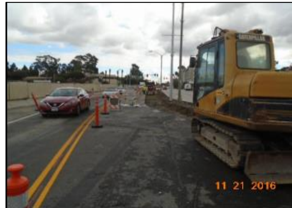
Powell graded island at Avalon and Carson.
