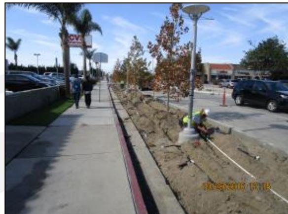
Installing irrigation laterals, risers, and heads in parkway
