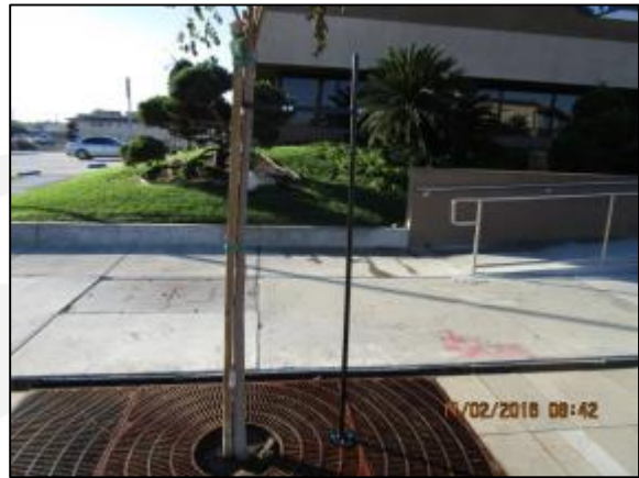
Tree stake installed.
