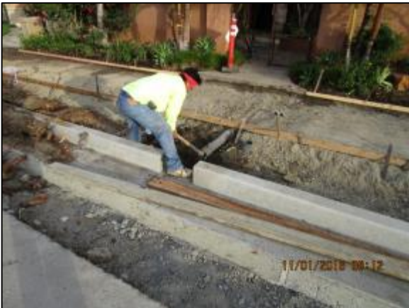
Placing sidewalk on north side of Carson.
