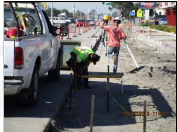
Checking form elevation.
