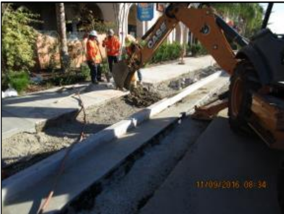
Doty Bros. relocating fire hydrant
