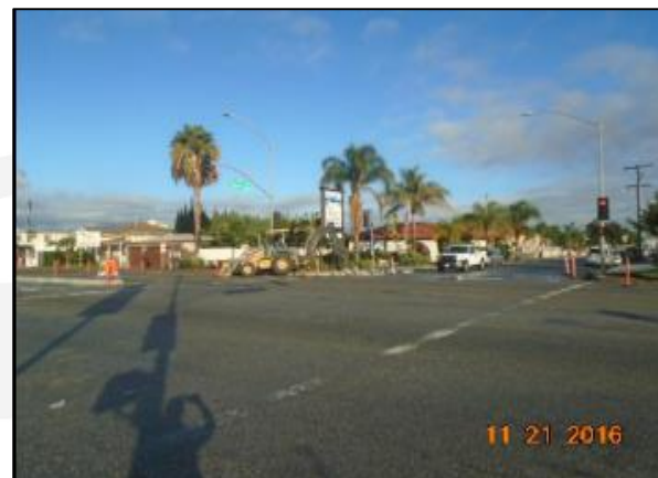
Demolition at north side Carson St. from Monetta to Figueroa.
