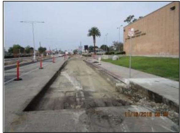
Cold milling north side of Carson.
