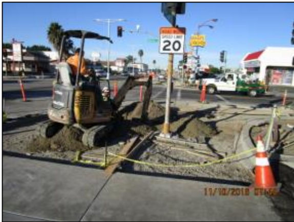
Excavating to locate water line.
