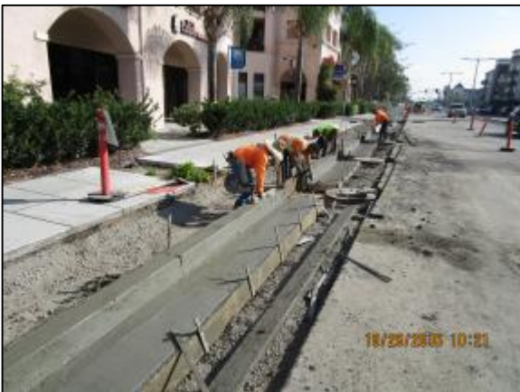
Finishing curb and gutter
