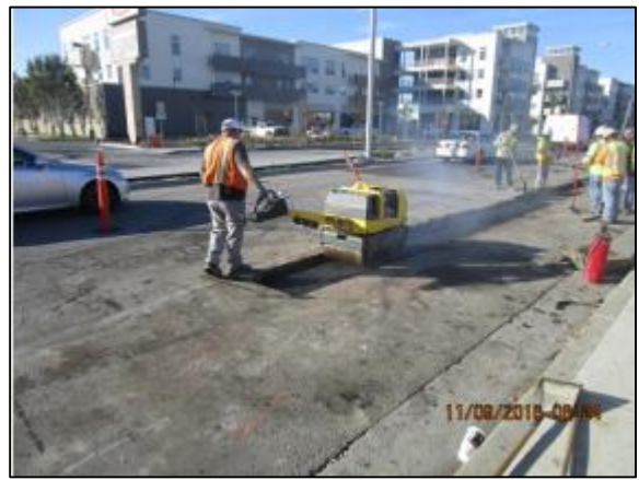
Paving Recycled water trench on Carson.
