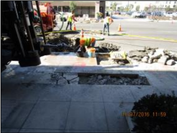
Potholing for directional boring.
