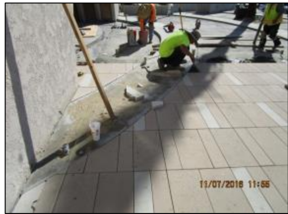
Installing architectural pavers at City Hall.
