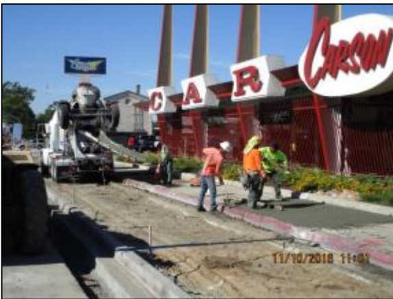
Placing sidewalk on north side of Carson.
