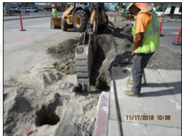
Trenching through slag north side east of Orrick.
