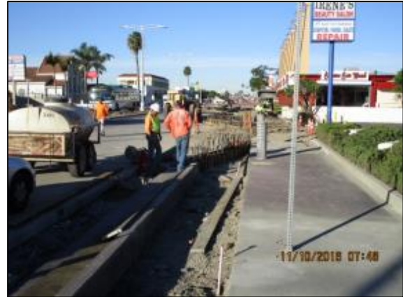
Forming curb and gutter.
