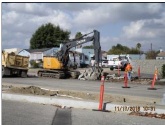
Demolition of sidewalk near Main.
