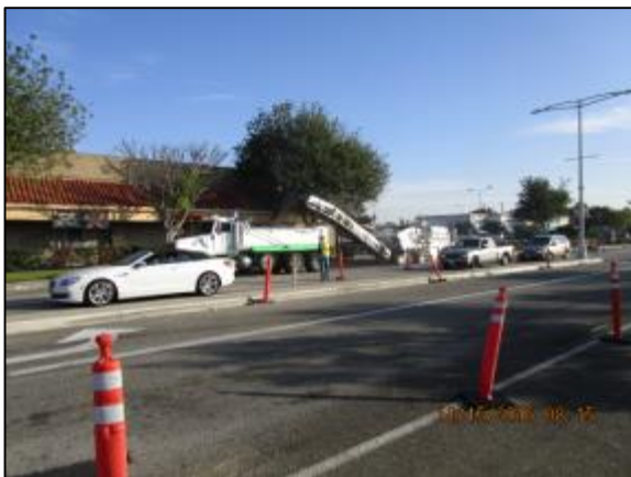
Cold milling AC on north side of Carson.
