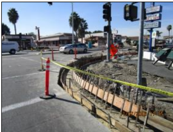
Curb return formed Carson at Dolores.
