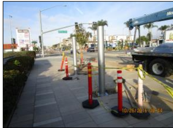
Bus Shelter supports installed
