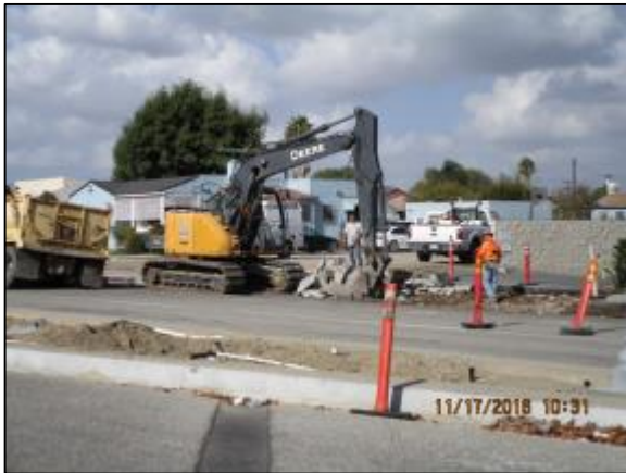
Demolition of sidewalk near Main.
