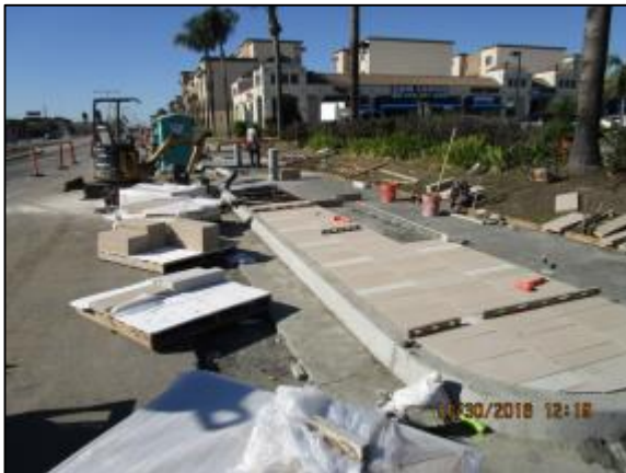
Installing pavers on north side just east of Grace.
