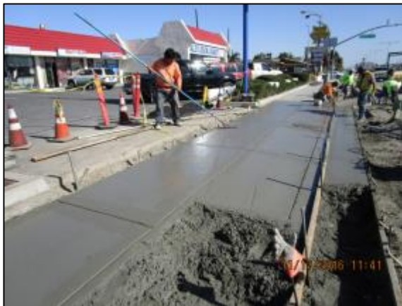
Finishing driveway north side of Carson.
