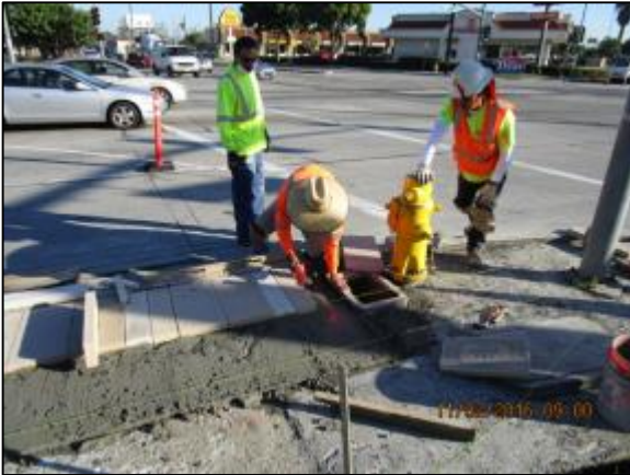
Placing pavers on south side of Carson west of Main.
