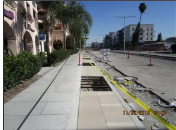
Tree grate frames installed.
