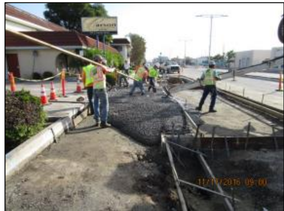
Placing driveway north side of Carson.
