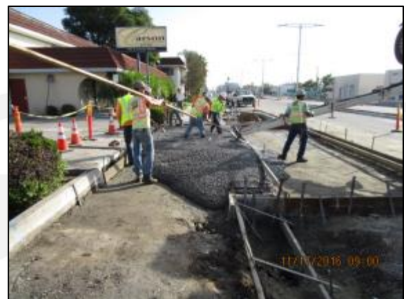
Placing driveway north side of Carson.
