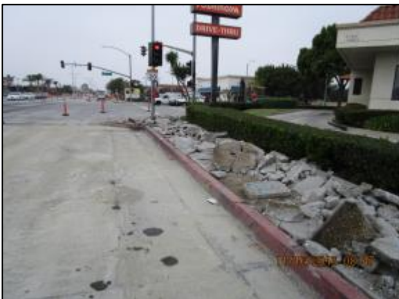
Demolition of sidewalk near Main.
