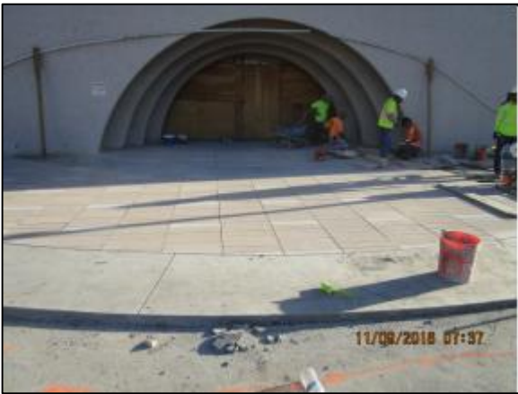
Installing pavers at City Hall
